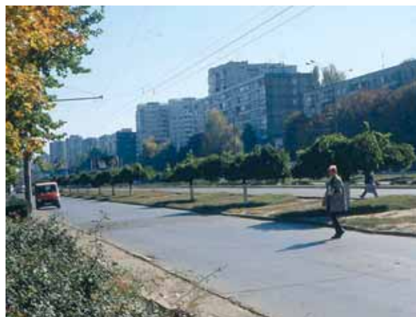
Public sector housing, Chisinau
