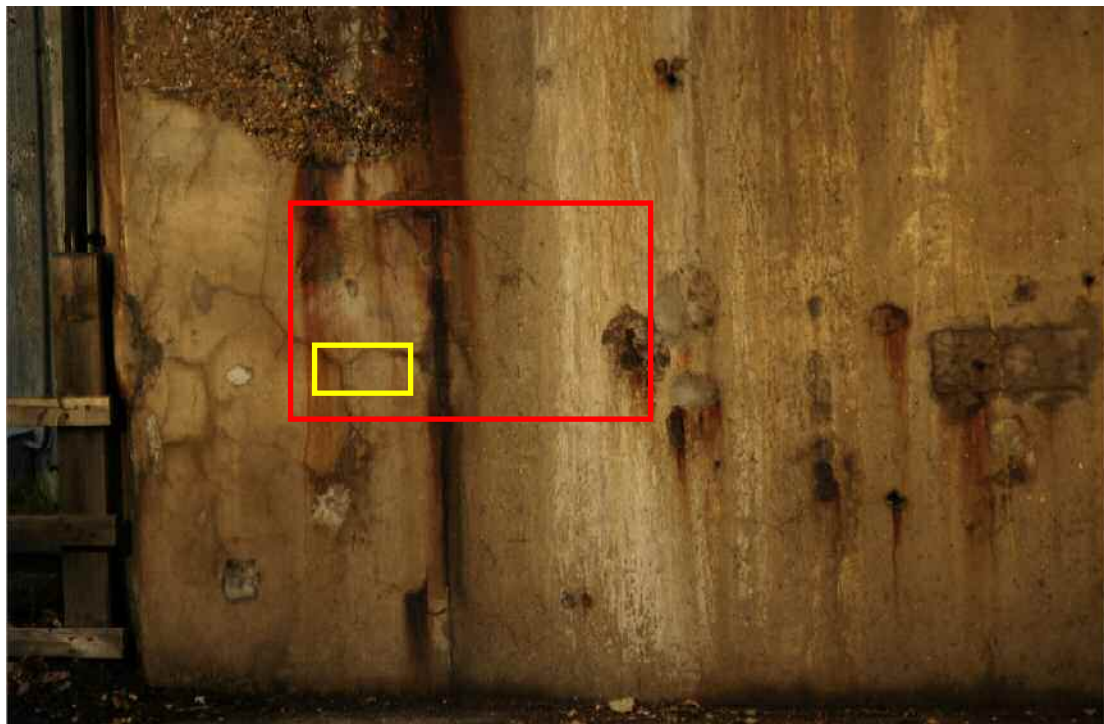
Figure 10: Full image of part of west internal wall
