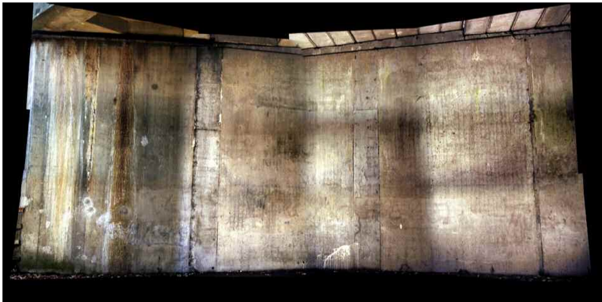
Figure 3: Single image from twelve overlapping images taken from two positions
