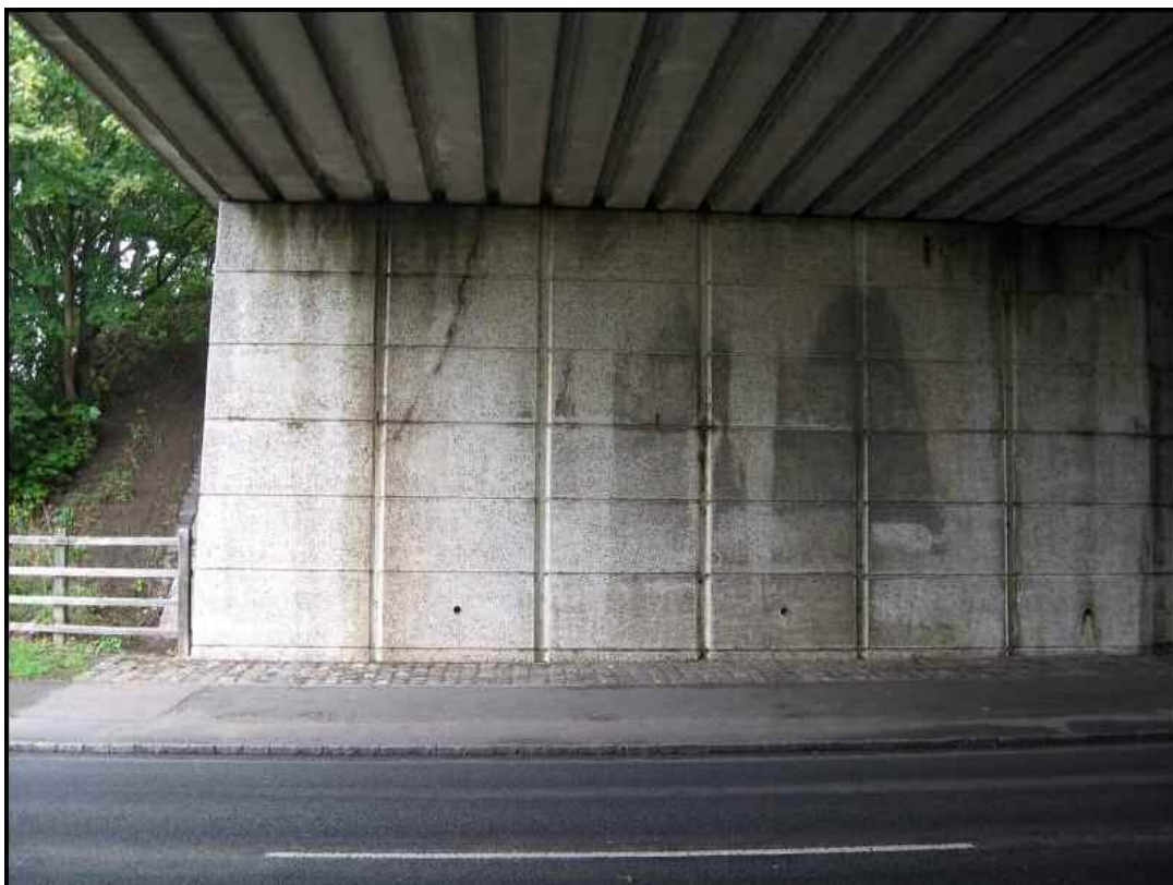
Figure 17: Eton Wick site. A332 over B3022.
