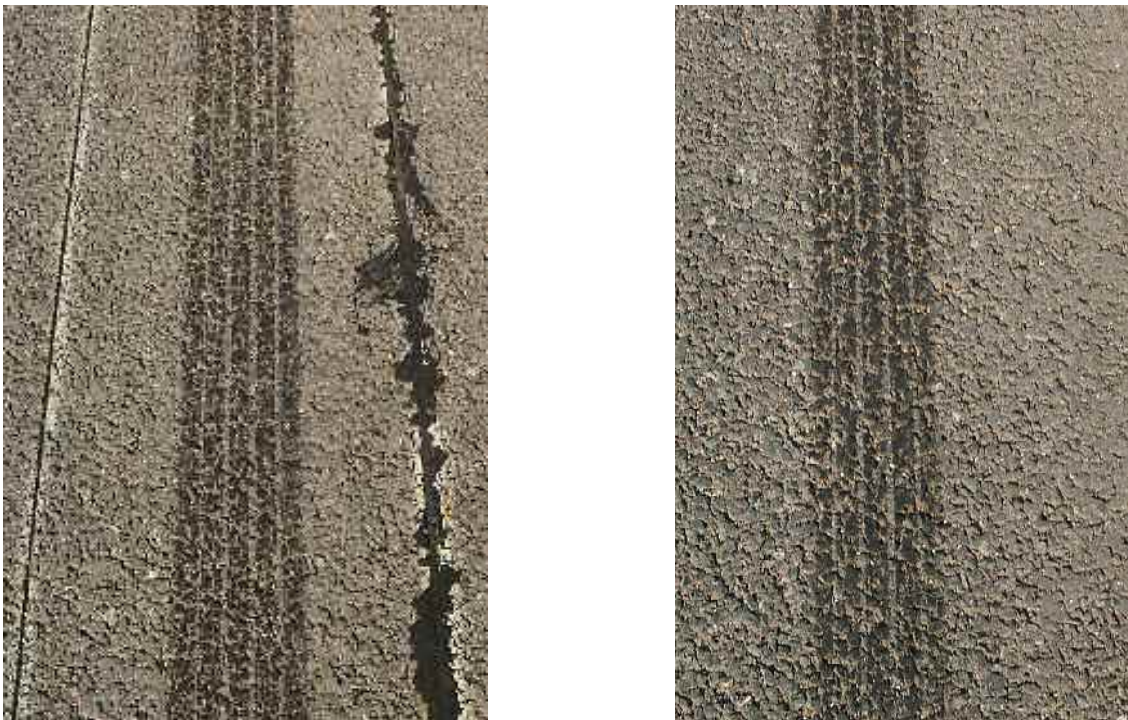
Figure 2.9. Low profile tyre, normal pressure (left) and +30% pressure (right)
