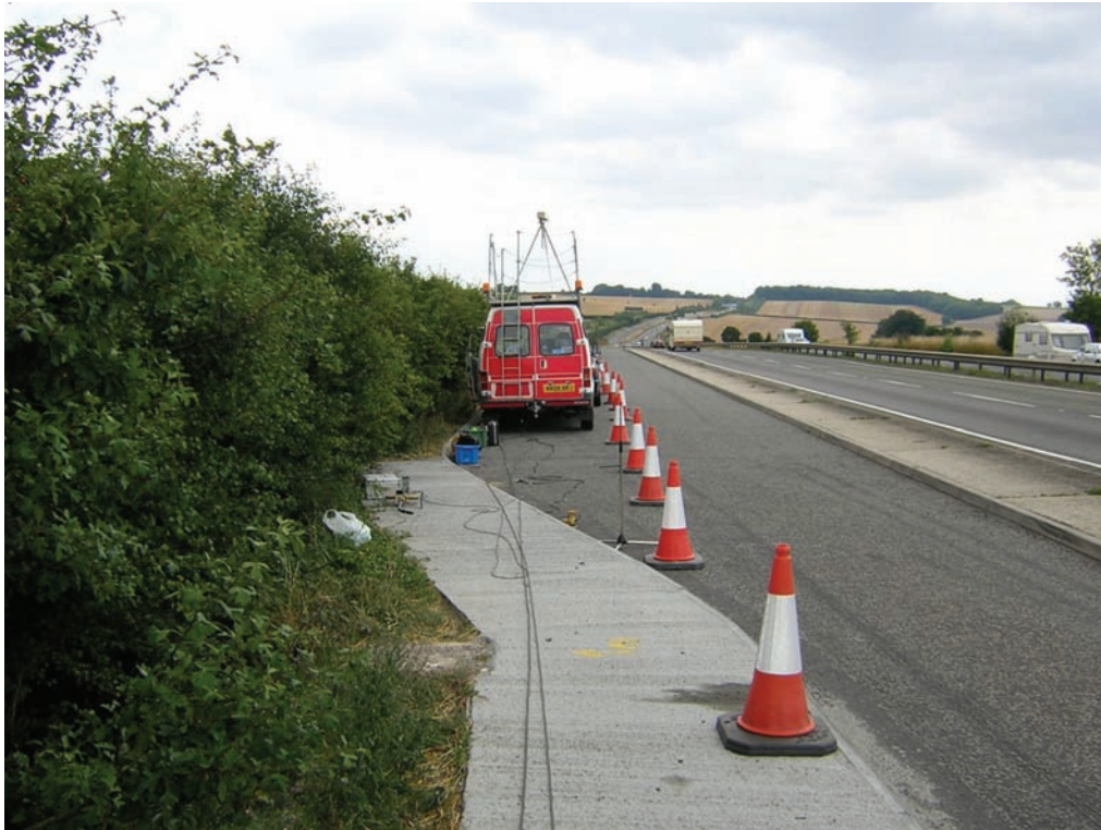
Figure 2.2: View of measurement set up at Site 2
