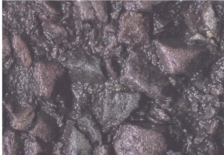
Figure 4.5 Example image from a damp portion of road surface (brightness altered for printing purposes)
