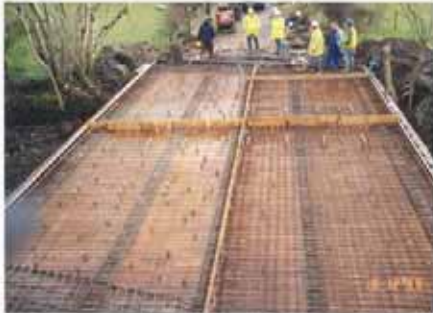
Photo 8: deck slab reinforcement
