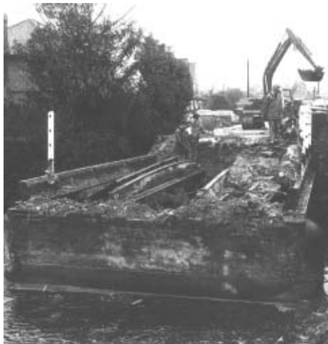
Figure 1 Demolition of the Hythe End bridge, from Daly and Raggett (1991)
