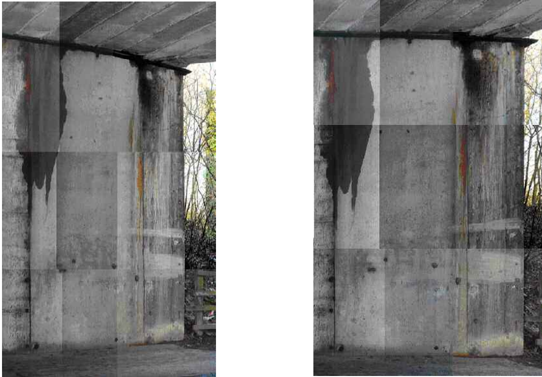
Figure 9: Example of images collected on site (left) and reprojected to appear perpendicular (right).
