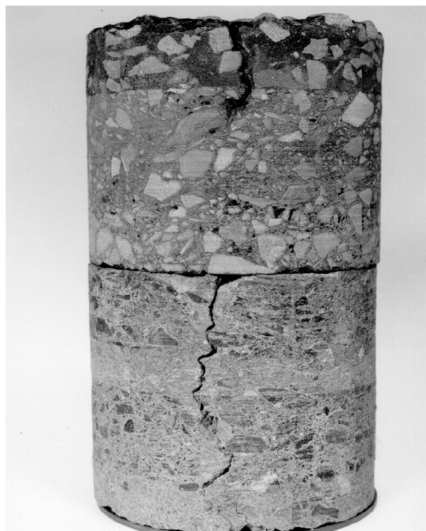
Figure 2. Core from a recently initiated reflection crack
